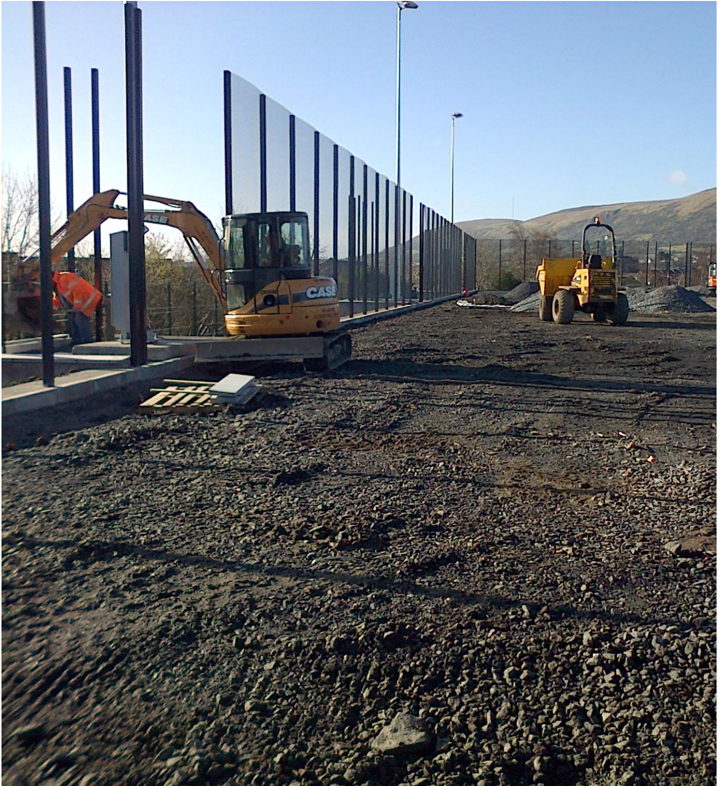
Construction underway (January 2014)
